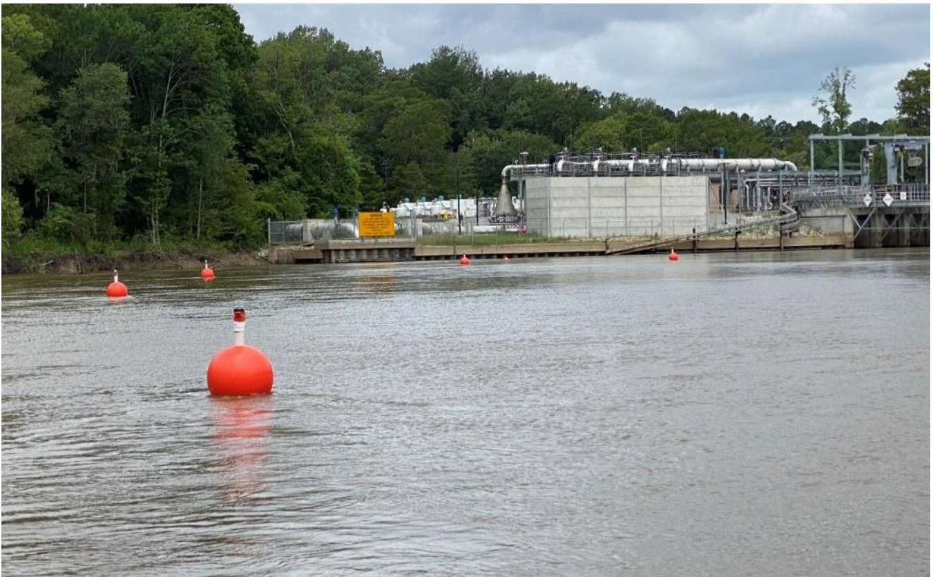
Figure 2-2 Upriver Semi-Permanent Buoys, Looking Toward Injection Plant
