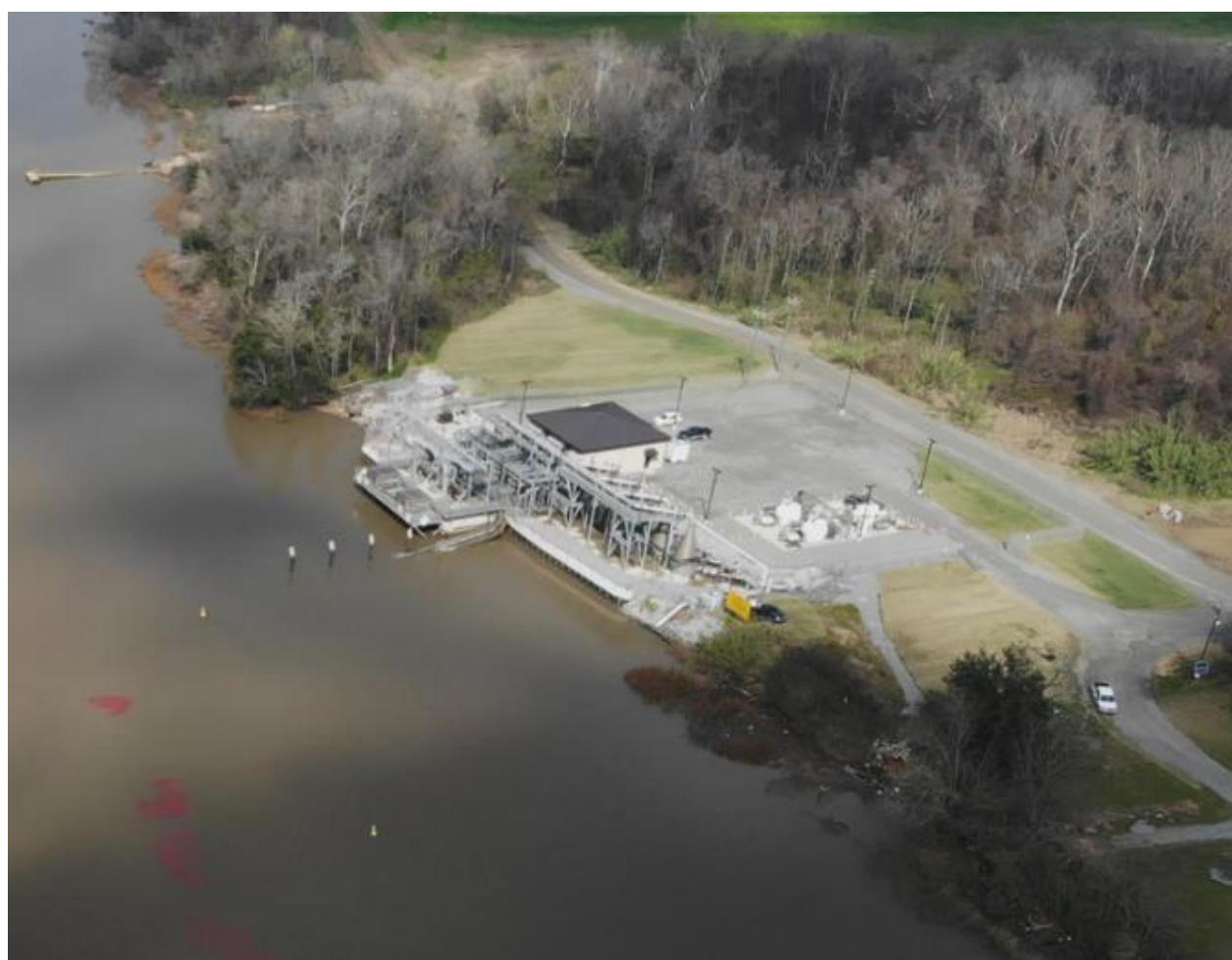
Figure 2-5 Dye Plume from Front River Diffuser Near Downriver Plant
