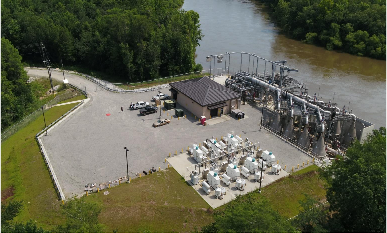
Figure 1-4 Upriver Oxygen Injection Plant
